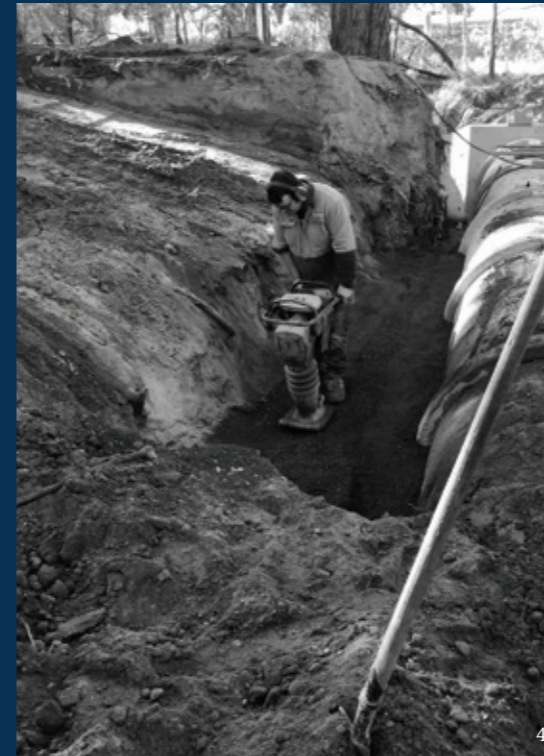
Major culvert renewal on Upton Rd
