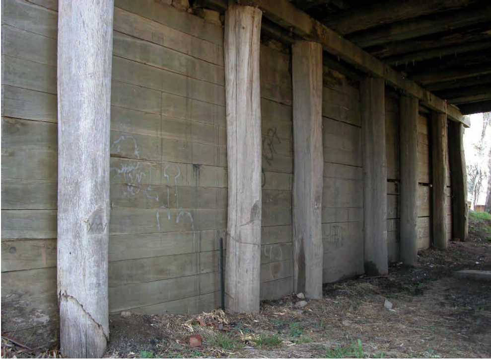
Timber piles in good condition.
