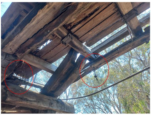
Image: Loose connections between cross-ties and deck. Source: Mim Butcher.
