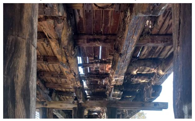
Image: Underside of bridge at northern end with two girders/stringers at centre. Note the natural cracking from drying process. Source: Mim Butcher.
