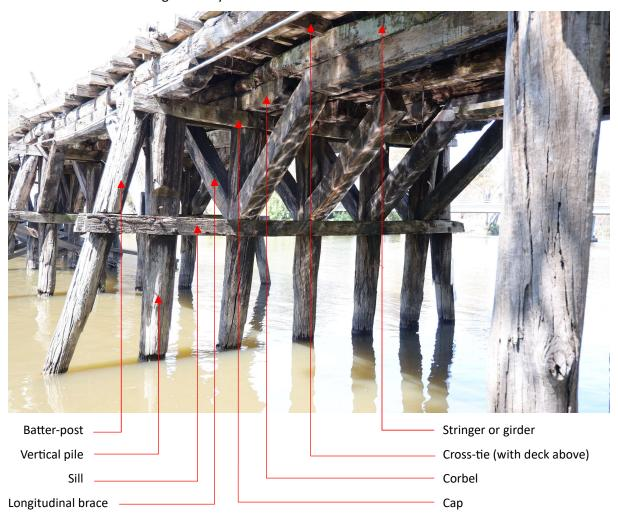
Image: View of underside of Chinamans Bridge with main bridge components indicated. Source: Thomas Cohen.
