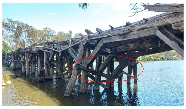
Image: Collapsed sill at southern end of bridge resulting in collapse of bracing connected to it. Source: Mim Butcher.
