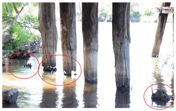
Image: View of piles in the northern-most bent showing two completely rotten through and two piles completely missing. Source: Thomas Cohen.
