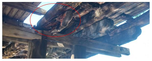
Image: Termite damaged corbel. Source: Mim Butcher.
