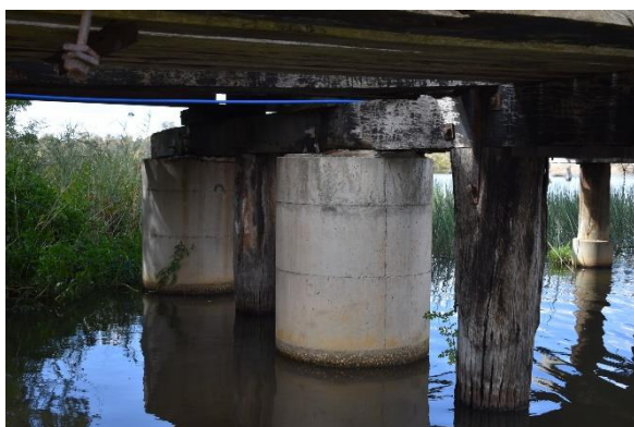
Figure 18. View of contemporary concrete piles on Kirwans Bridge. Source: Extent Heritage, 2022.
