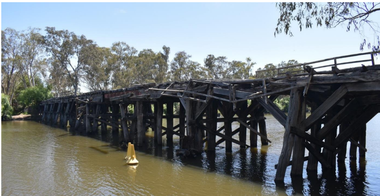
Figure 9. Chinamans Bridge, looking north. Source: Extent Heritage, November 2023.
