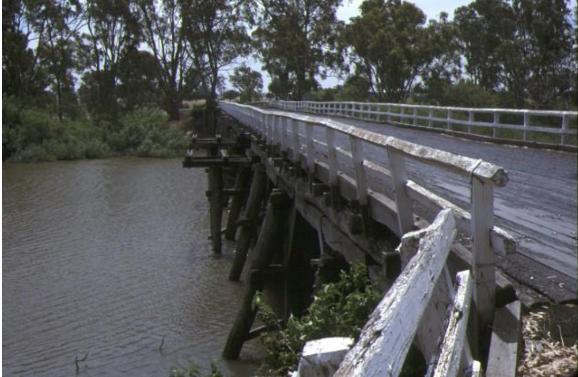
Figure 7. Chinamans Bridge. Source: National Trust of Australia (Victoria), 1987.
