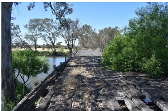
Figure 10. View of the bridge decking looking southeast. Source: Extent Heritage, 2023.
