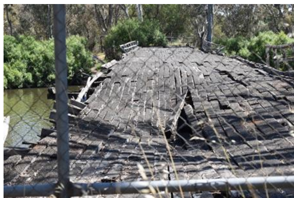
Figure 11. View of the bridge decking looking northwest. Source: Extent Heritage, 2023.
