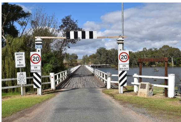
Figure 16. Direct overview of Kirwans Bridge looking south. Source: Extent Heritage, 2022.
