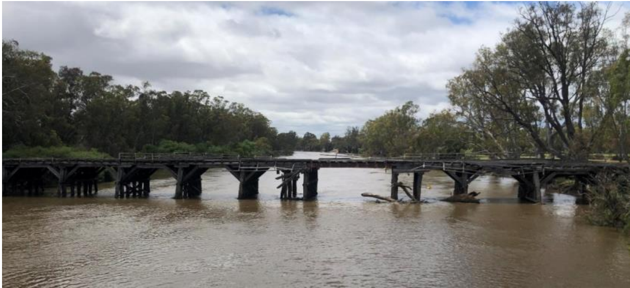
Figure 15. Overview of the structure. Source: Jo Lyngcoln, Heritage Victoria, November 2022.
