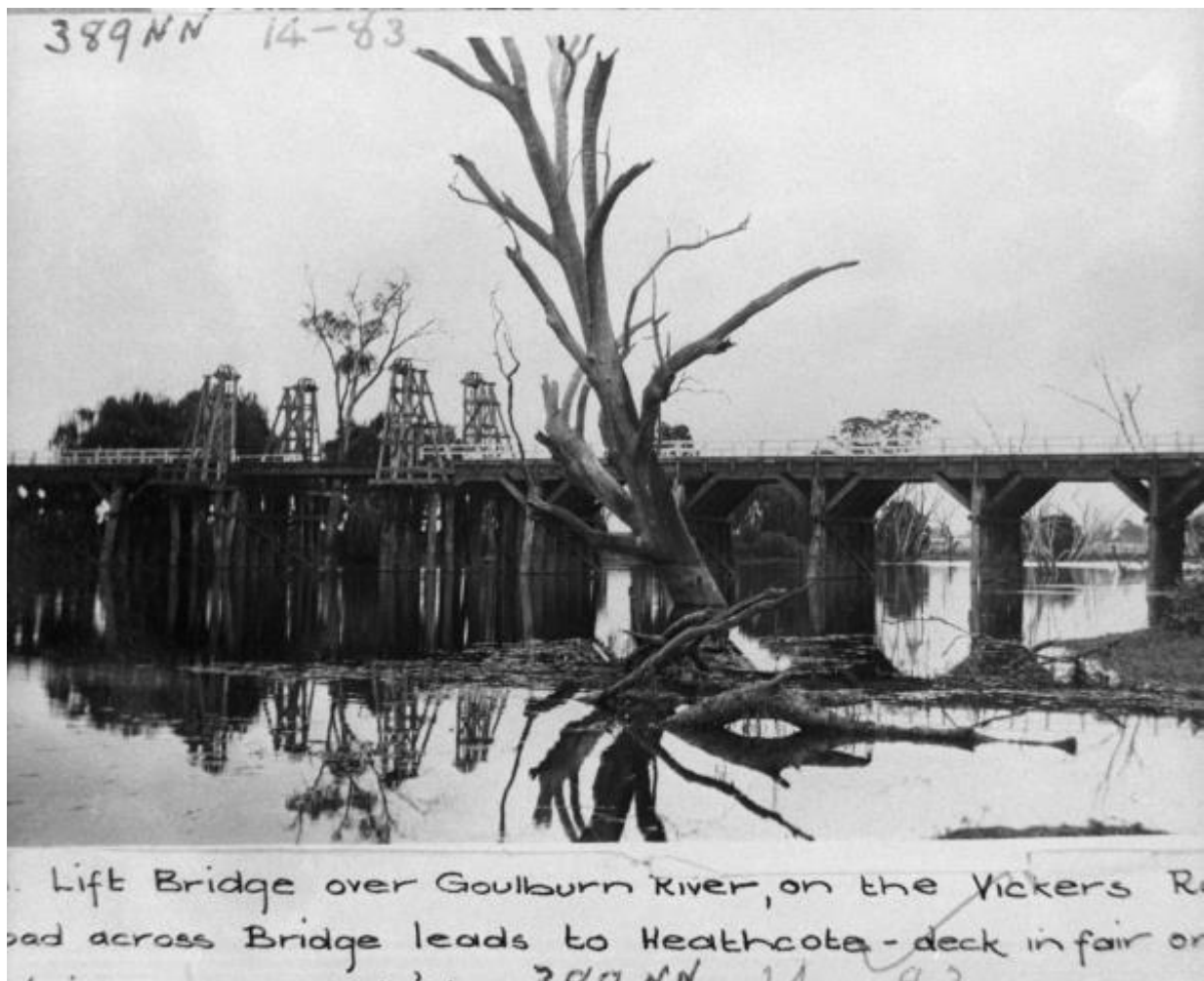
Figure 5. Lift Bridge over Goulburn River, Vickers Road. Caption reads "deck in fair order". Source: PROV, VPRS 17684/P0003/212, Negative number 14_00083, 1 April 1914.
