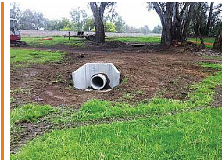
DRAINAGE IMPROVEMENT WORKS IN VIOLET TOWN
