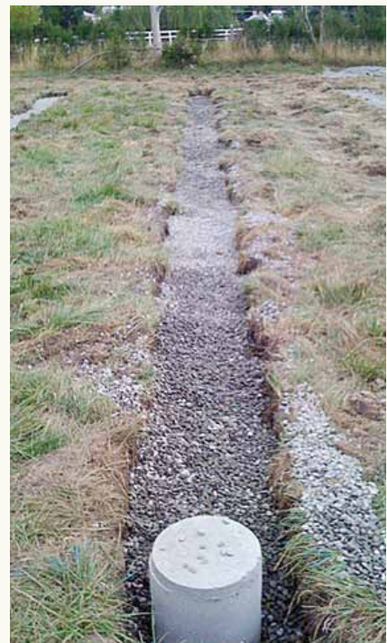
INSTALLATION OF ABSORPTION TRENCHES AS PART OF ALL WASTE SEPTIC SYSTEMS.
