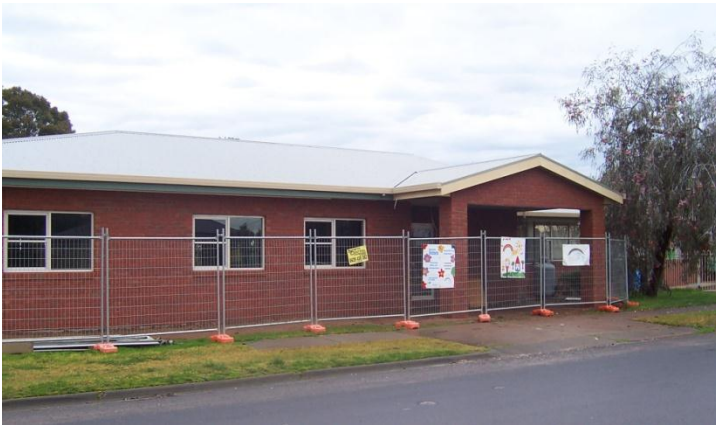
Works underway at the Nagambie Pre-School
