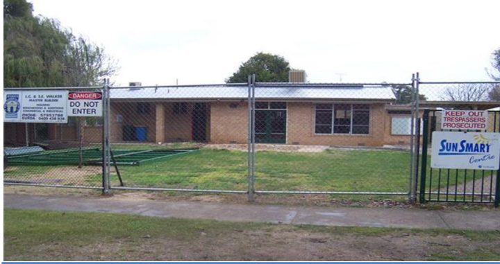
Works underway at Euroa Pre-School
