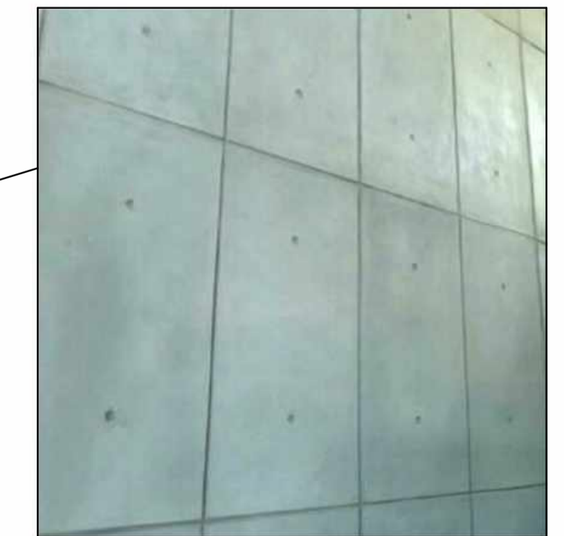
Precast Concrete Wall Panels
