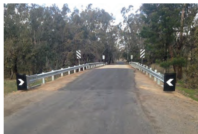
Local Bridge Maintenance
