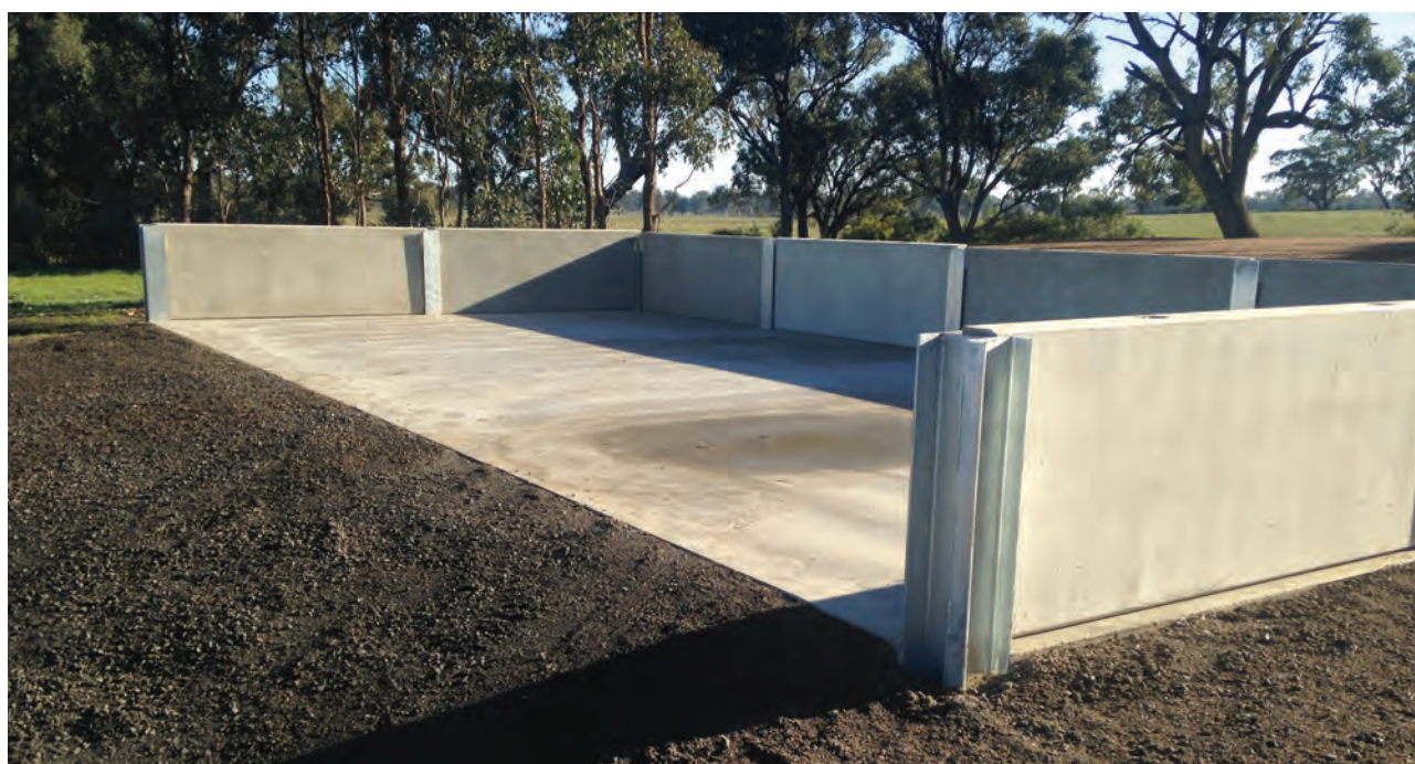
Concrete bay to house scrap metal ~ Nagambie Transfer Station
