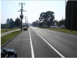
The construction of the freeway bypass creates an opportunity to reconsider how High Street will work as a traditional 'Main Street' through a country town
