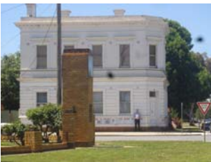
The old two storey Bank Building in High Street is approximately 10.5 metres tall. This is roughly the equivalent of a modern-day three storey building
