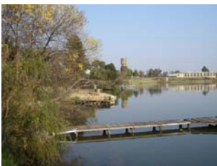
Many private jetties protrude into Lake Nagambie. Some are in poor condition and might present a liability hazard.
