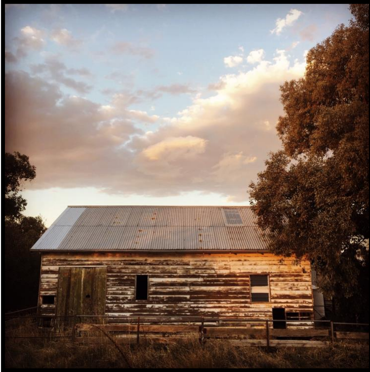
19 th Century shearing shed, repaired & adapted to 21 st Century work shed, Sheans Creek. Image: C. Hammond 2018
