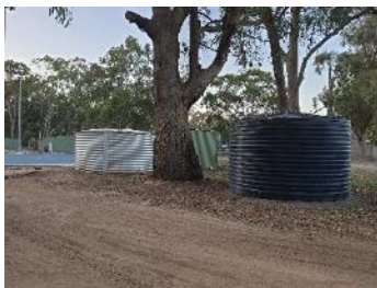
Figure 13 – Above Ground Tanks
