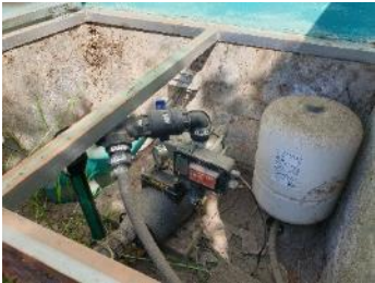
Figure 35 – Groundwater Pump and Pressure Tank
