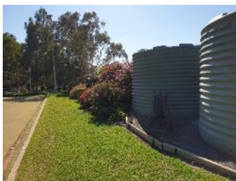
Figure 19 – Above Ground Tanks - Plastic
