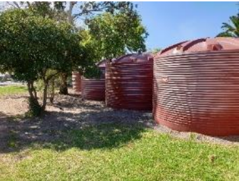
Figure 36 – Above Ground Tanks
