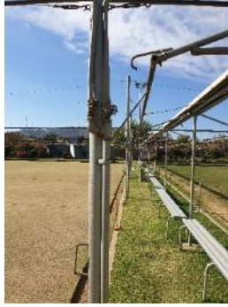
Figure 23 – Manual Irrigation System
