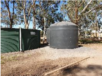
Figure 10 – 2No. 20,000L Plastic Tanks
