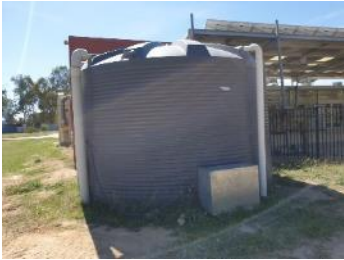
Figure 40 – Existing Rainwater Tank
