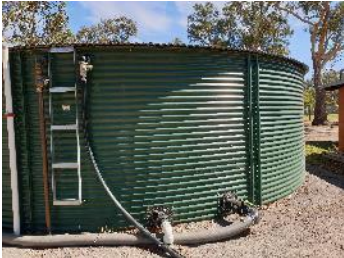
Figure 5 – 100,000L Steel Tank
