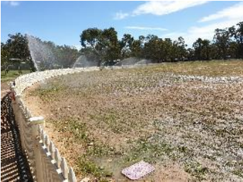
Figure 6– Pop-up Sprinkler System
