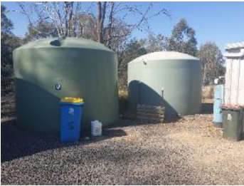
Figure 30– Above Ground Tanks
