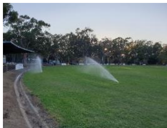
Figure 14– Pop-up Sprinkler System
