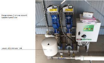
Figure 7– Pumps, Filter and Pressure Tank
