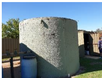
Figure 20– Above Ground Tank - Concrete
