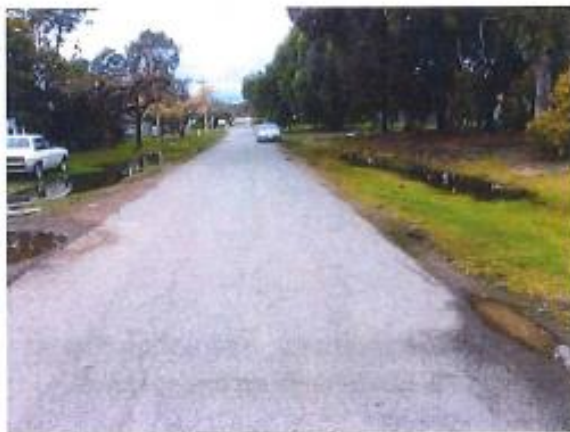
PHOTO 1 Rowe Street - conditions pre-construction
