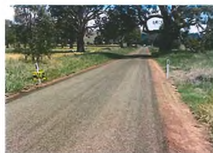
ROAD PAVEMENT REHABILITATION
