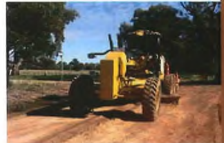
GRAVEL ROAD RE-SHEETING
