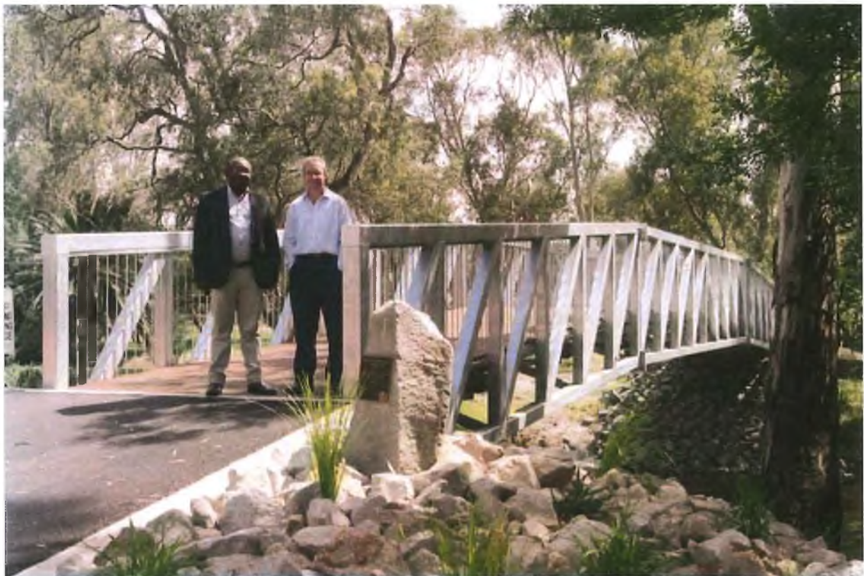
PETERSON ASANTE (L) AND JOHN OWEN (R) ON "EUROA'S LITTLE HARBOUR BRIDGE" CONSTRUCTED AT THE EUROA CARAVAN PARK
