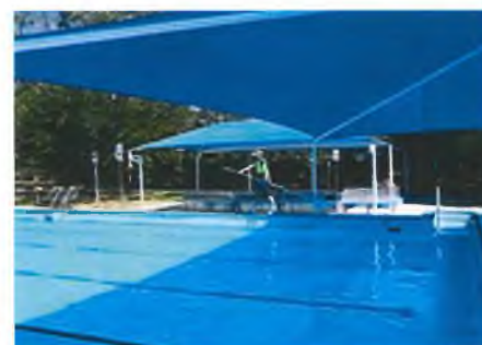
SWIMMING POOL REFURBISHMENT
